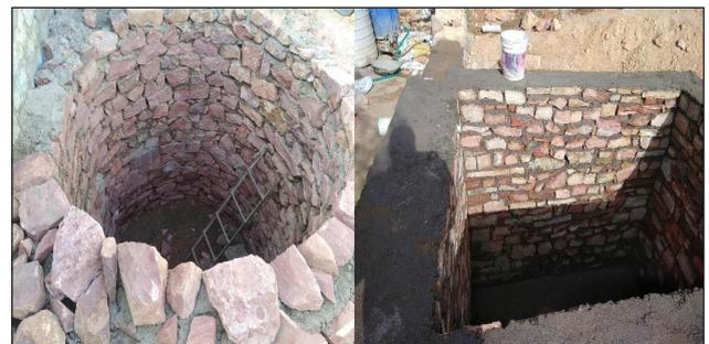
**Fig. 1:** A typical picture of round and rectangle shaped Tanka
